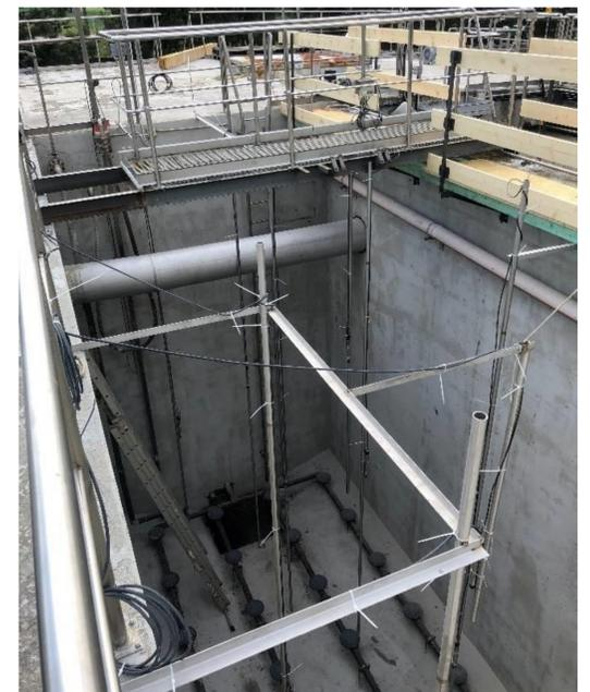
Figure 2. Tank with footbridges and the fixed probes.
